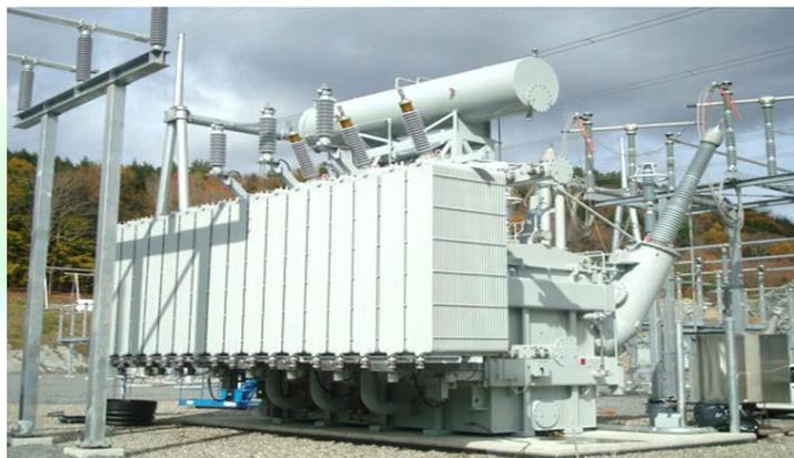
**400kV/115kV 200MVA(周溫負50°C)**
