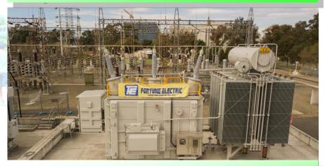
Ultra-Low Noise 132kV 45MVA Power Transformer to Australia
