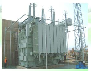
220kV 210MVA 11 Units Power Transformer to Peru
