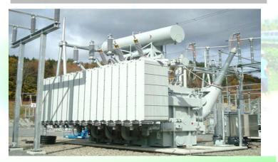
400kV/115kV 200MVA Transformer to America(ambient temperature - 50 °C)
