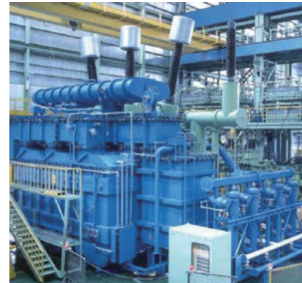
▲ Oil type power transformer for hydropower generator
