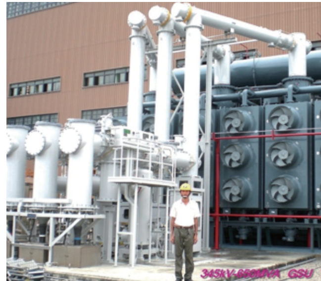
▲ Oil type power transformer for thermal power generator
