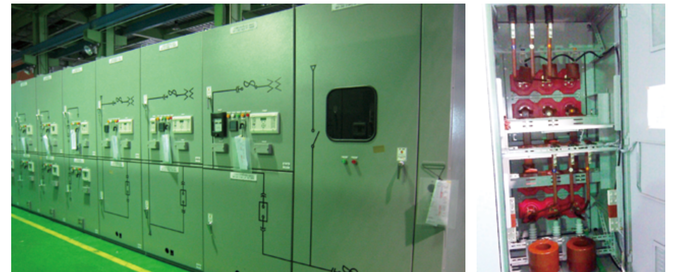
▲ Metal lock type switchgear
